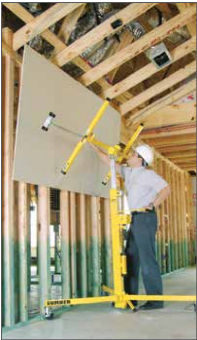
Steering leveler provides optimum positioning.
